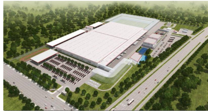
New factory under construction
